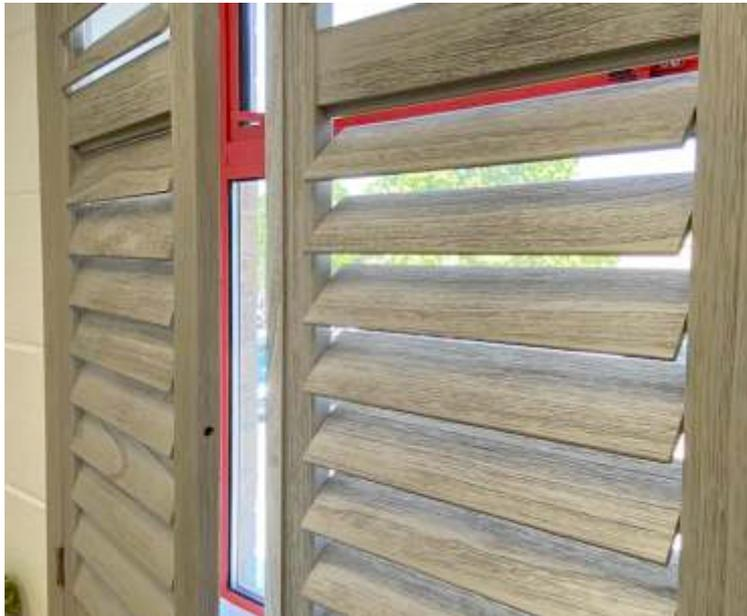
Over time, it is possible that the slats can lose tension. This is nothing to worry about as you can adjust them using the slat tension screws which are to be found in the inside edge of the panels. A quarter turn of the screw is sufficient.
